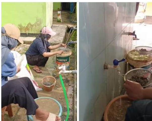
Gambar 8. Pembersihan Media Filter
