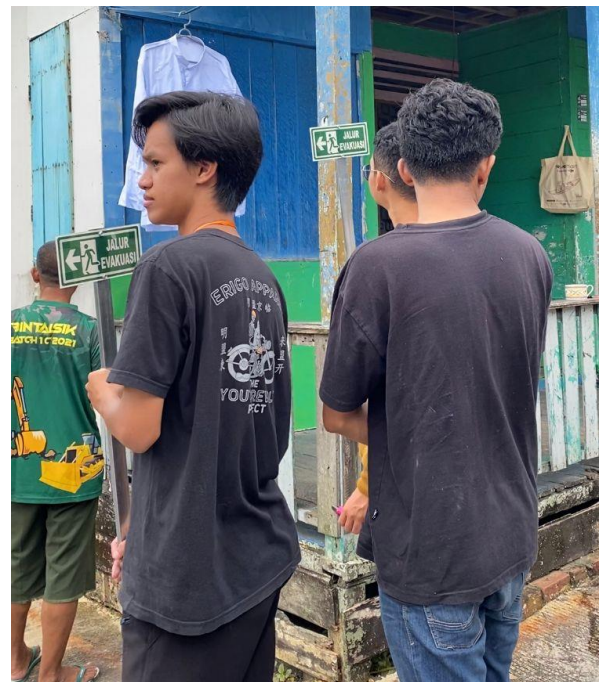
Gambar 1. Proses pemasangan safety sign
